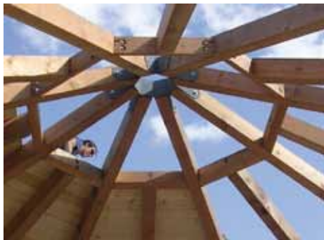
Mitchell Park Bandstand Construction
